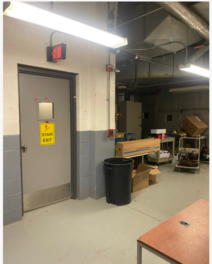
Figure 5. The basement of the math building was listed on the campus map as including a universal restroom, but its location was unclear and the basement felt like it was not a public space.
