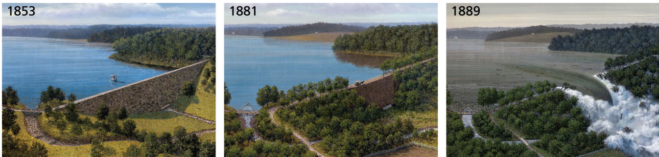
Figure 1. Johnstown Flood National Memorial, Pennsylvania. The South Fork Dam as it appeared when newly constructed (left), in a state of disrepair (middle), and breaching (right). Art by L. Kenneth Townsend.
