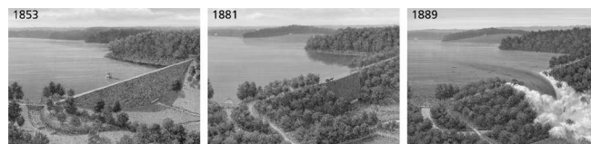
Figure 1. Johnstown Flood National Memorial, Pennsylvania. The South Fork Dam as it appeared when newly constructed (left), in a state of disrepair (middle), and breaching (right). Art by L. Kenneth Townsend. (see page 96 for full color version)
