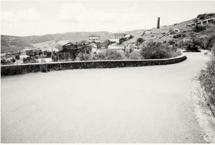
Figure 13. Road from Carbonia to Iglesias.
